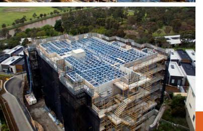
Although timber has served us well for many years, builders and project managers are now finding that the durability, strength and longevity of cold-formed steel frames and trusses make them the ideal material for multi-residential projects.
